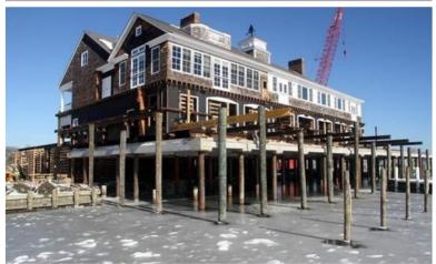
Figure 2: This image was taken during the elevation of the Bay Head Yacht Club, an historic structure, after it was substantially damaged during Superstorm Sandy.
